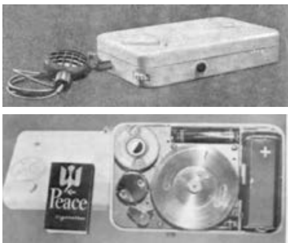
Fig. 5.15. External and internal views of the Minifon (1952) (16)
