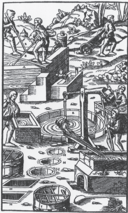
Figure 2.1 Manufacture of Alum (G. Agricola, De Re Metallica , Dover, p. 567) 5,6
