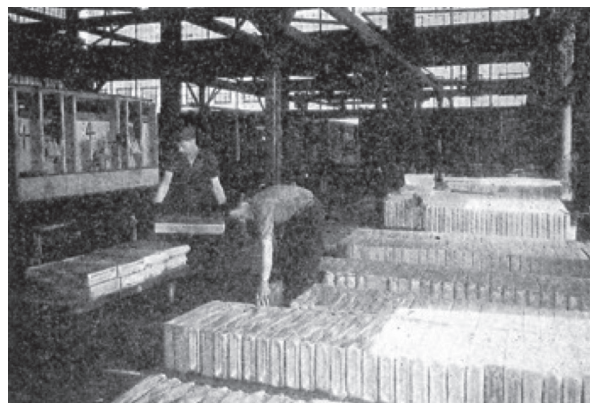
Figure 3.7 Alcoa Foundry Casting Ingots for Sheets 17
