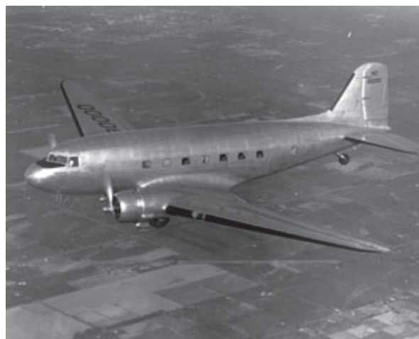
Figure 4.18 DC-3 Using Alcoa's Alclad 24S-T3 for Fuselage Skin 62
