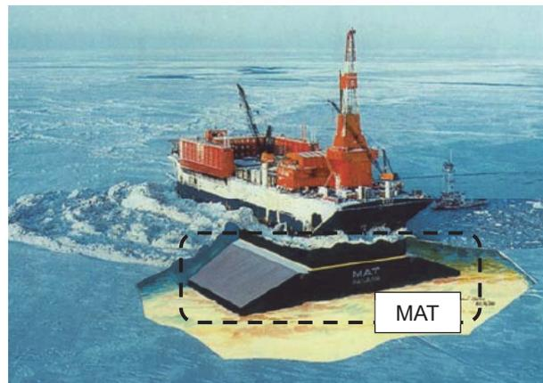
Fig. 8.10 Typical installation, MAT/SSDC in ice-covered seas: Significantly reduced seabed preparation work + Improved resistance to ice forces from drifting ice.<sup>8-1)</sup>
