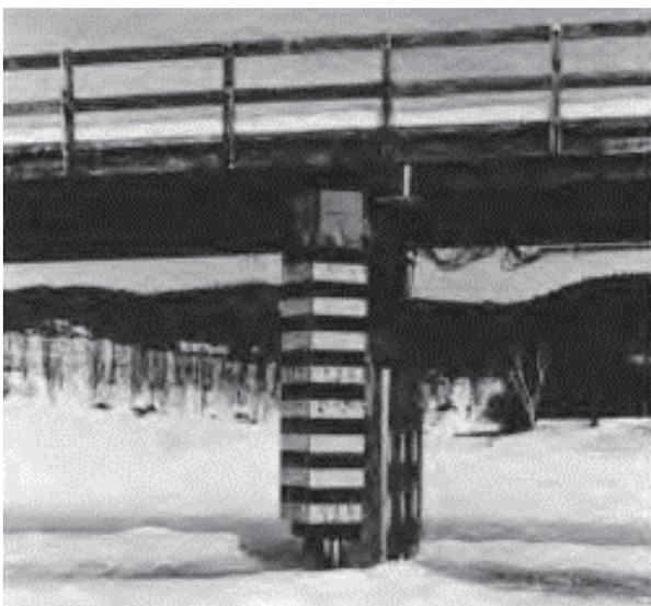
b) In situ tests: River pier width 600 mm.<sup>7-1)</sup>
