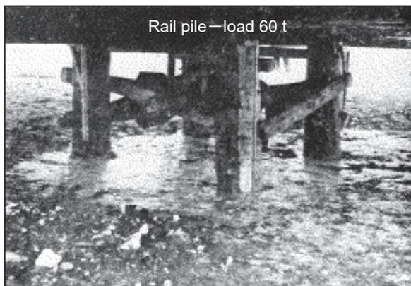
Fig. 4.10 Ice sheet-rail pile load test, photograph: Test table (four pine log legs, each 30 cm diameter) with 60 t load placed on ice sheet (70 cm thick)—Examined amount of subsidence and the condition of cracks in the ice sheet.<sup>4-6)</sup>
