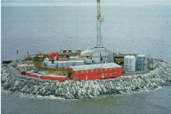
Fig. 8.4 Earth-filled artificial island, Beaufort Sea, constructed late 1970s, photograph: Structure surrounded by sandbags to withstand external forces from waves and sea ice.<sup>8-1)</sup>
