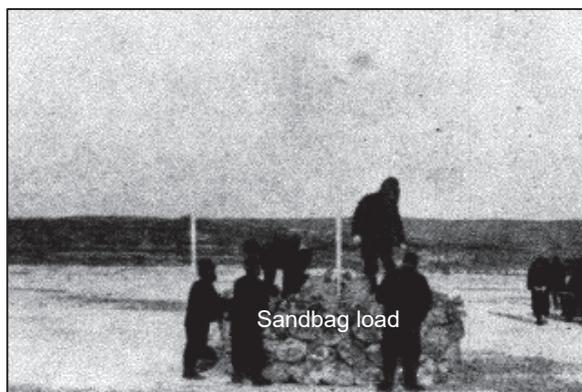
Fig. 4.9 Ice sheet sandbag load test (in situ), photograph: Examined effect of load weight (max. load 40 t) and loading time (4-8 hours) on naturally frozen ice sheets with thicknesses of 34-98 cm—sandbags (30 kg each).<sup>4-6)</sup>
