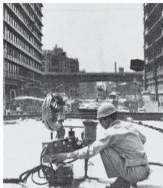
(c) 鋼床板の現場溶接
