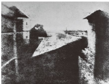
Photograph 2-1 View from the Window at Le Gras 2)
