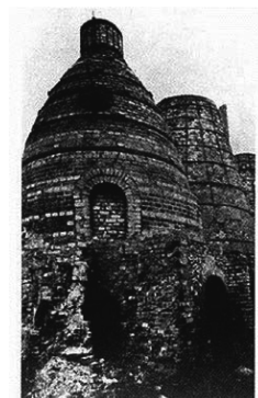
Fig. 2.2 A Shaft Kiln built by Aspdin 1)
