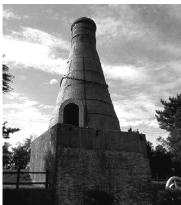
Fig. 2.8 Shaft Kiln (Bottle Kiln) Still Standing at the Taiheiyo Cement Corporation Onoda Plant 7)
