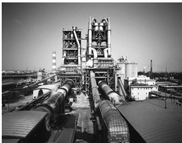
Fig. 1.4 Preheater Tower and Rotary Kiln 2)
