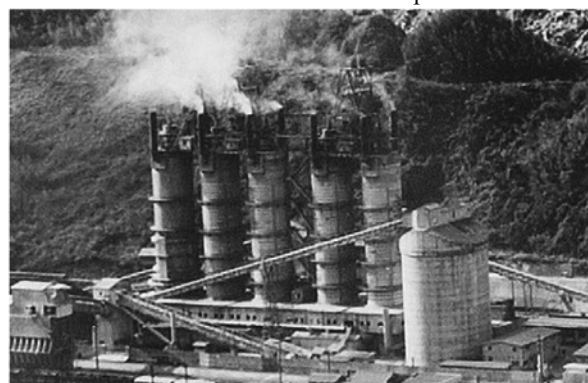
Fig. 4.7 Limekilns for the New Calcined Lime Process 7)
