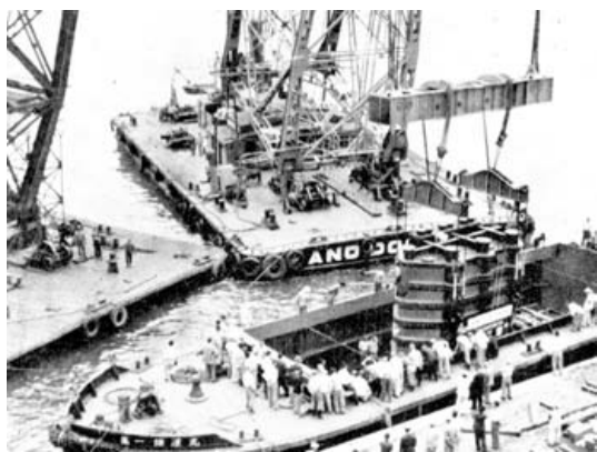
Photo 4.7. A 160MVA Transformer for the Tokyo Electric Power Company Chiba Power Station Shipped with the Use of a Floating Crane (1956)
