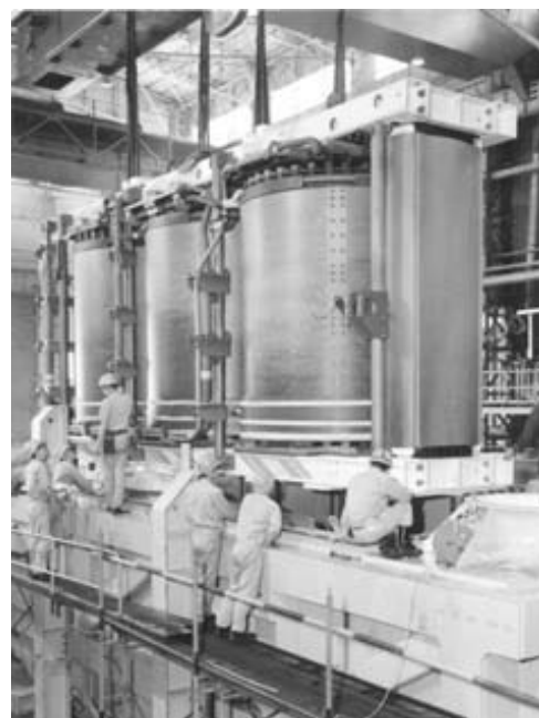
Photo 4.20. Core and Coil of the Shin-Koga Substation 1000/3MVA Transformer
