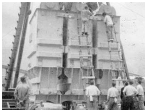
Photo 4.4. The First Special Three Phase Transformer, a 93MVA Transformer for the Electric Power Development Company Sakuma Power Station (1955, made by Mitsubishi)
