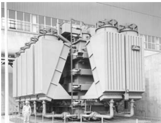
Photo 4.12. A 680MVA Transformer for the Tokyo Electric Power Company Anegasaki Power Station (1966, made by Toshiba)
