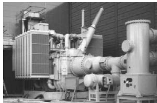
Photo 6.2. A 161kV, 68MVA, Low-Pressure Gas-Insulated Transformer for the Tohoku Electric Power Company Yanaizu-Nishiyama Geothermal Power Station (1994, made by Toshiba)
